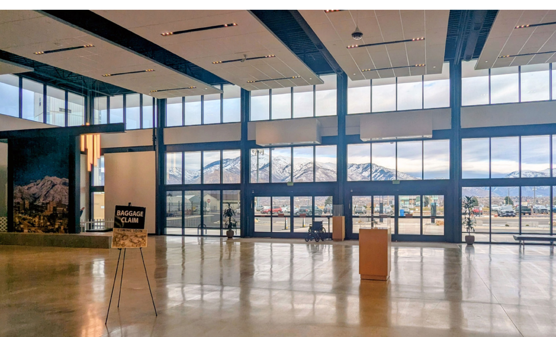
New terminal expansion at the Ogden-Hinckley Airport
