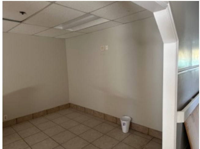
PHOTO 2: Asbestos Containing Wall System contains 4% Chrysotile Asbestos
