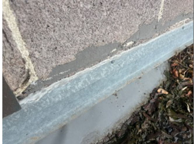
PHOTO 4: Light Grey Brick Sealant (5% Asbestos) and White Mortar (Trace % Asbestos)
