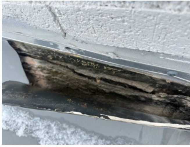
PHOTO 5: Black Roofing Skirt Tar contains 12% Chrysotile Asbestos
