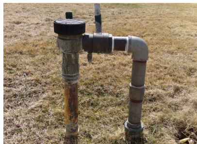
Pressure Vacuum Breaker (PVB)
