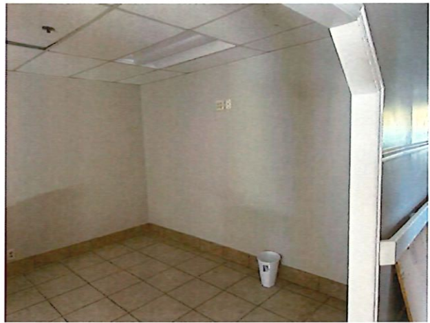
PHOTO 2: Asbestos Containing Wall System (Surfacing)
