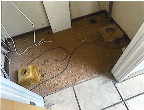
PHOTO 3: Asbestos Containing Rolled Vinyl Flooring
