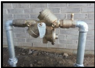
Reduced Pressure Principle Assembly (RP)
