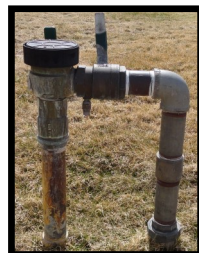
Pressure Vacuum Breaker (PVB)
