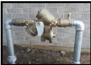
Reduced Pressure Principle Assembly (RP)
