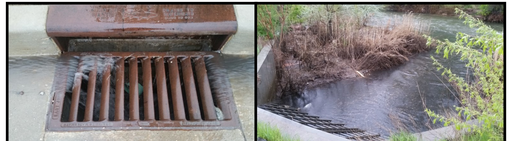
Storm water flows through storm drains directly to local creeks and rivers with NO TREATMENT.
