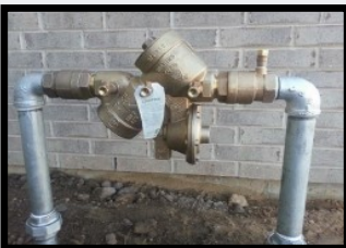
Reduced Pressure Principle Assembly (RP)
