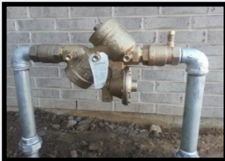
Reduced Pressure Principle Assembly (RP)
