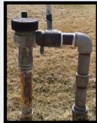
Pressure Vacuum Breaker (PVB)
