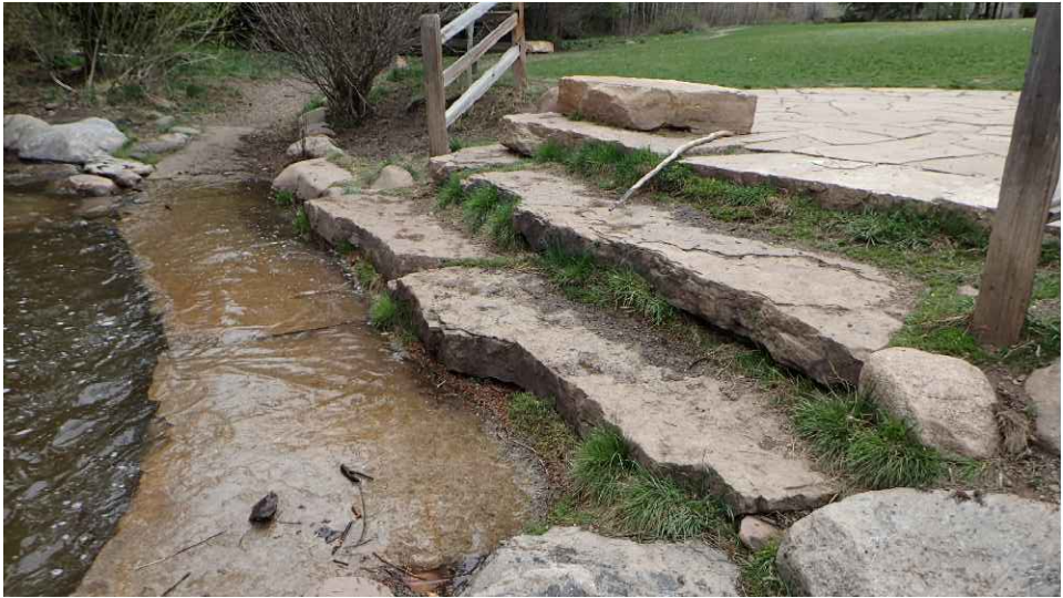
EXAMPLE PHOTO OF FINISHED SLAB STONE ACCESS STEPS
