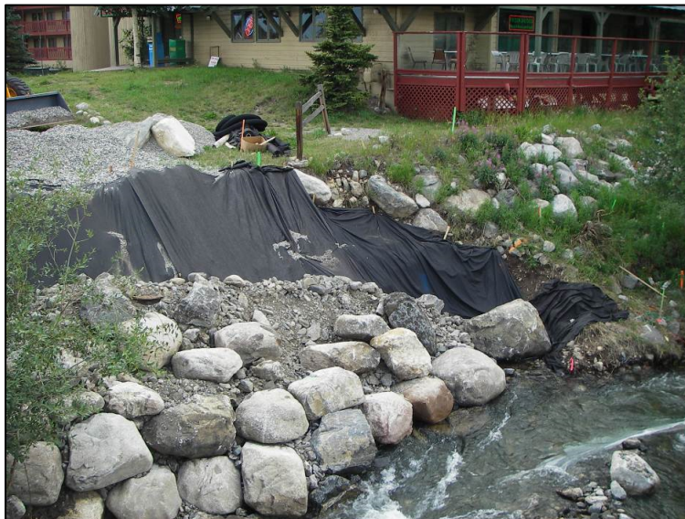
Figure 4.5. Filter fabric installation example
