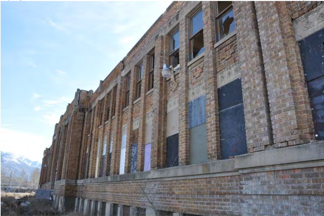
Photograph 7 of 13 North elevation. Camera facing southeast.
