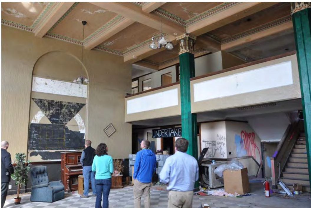
Photograph 10 of 13 Lobby interior. Camera facing northwest.
