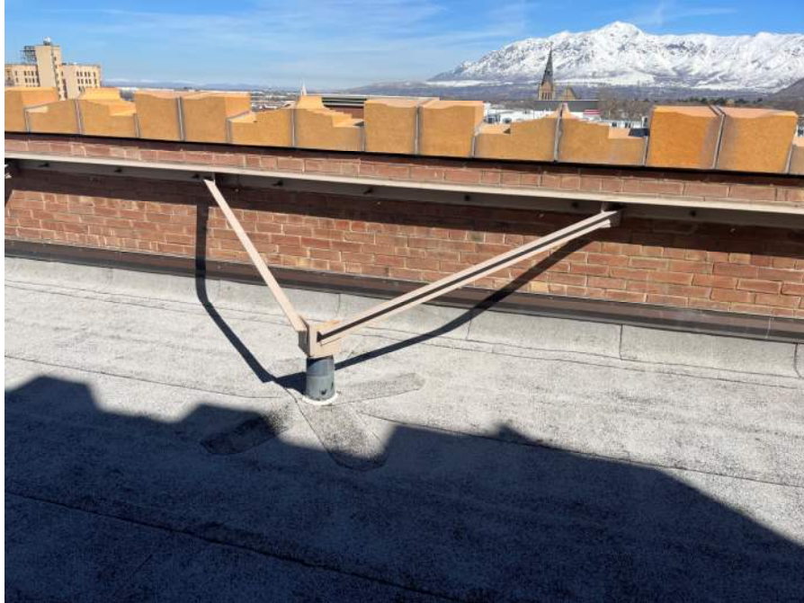
Photo 2 – Unreinforced masonry parapets braced back to roof diaphragm
