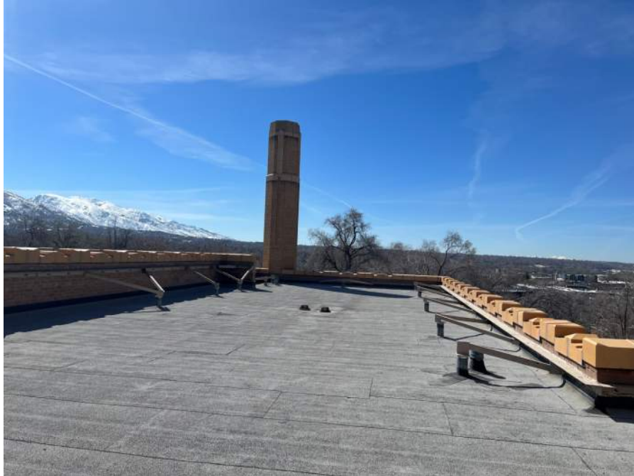
Photo 4 – Unreinforced masonry chimney
