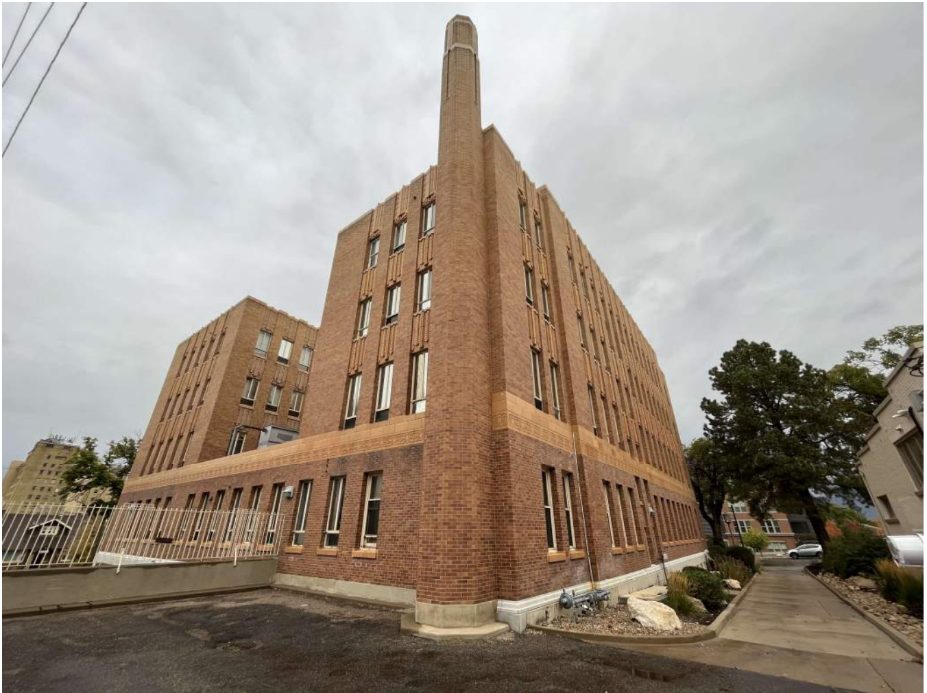
Photo 1 – View of unreinforced masonry chimney from southeast corner of building. Picture is taken from parking surface on top of basement wing.
