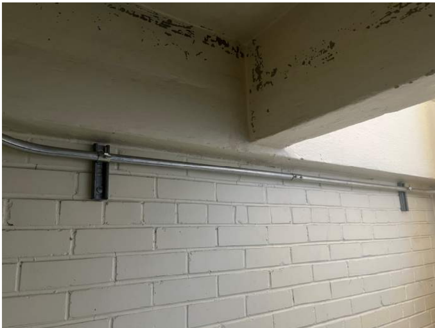
Photo 3 – Unreinforced masonry infill walls at concrete-frame
