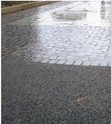
Porous paving surfaces reduce water runoff
