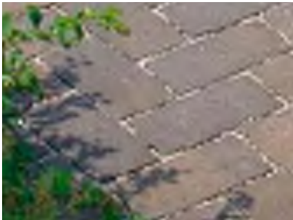
Brick pavers, when installed properly, can last as long as concrete and are also ADA compliant
