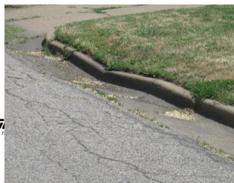
Damaged Curb and Gutter
