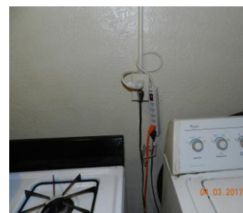
Inadequate electrical connections
